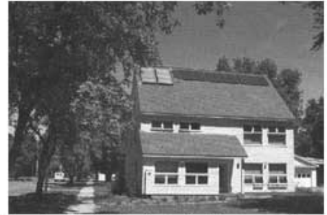
Figure 1 - The Hanson House includes two roof-mounted solar thermal panel and 12 photovoltaic modules with a peak rating of 1,440 watts.
